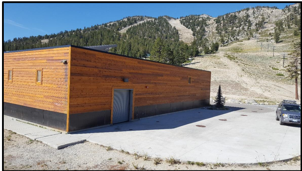
View of existing Winters Creek Lodge to the southwest.
