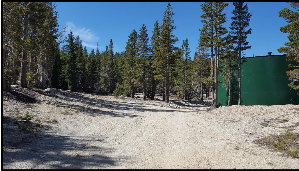
View to the south west toward proposed tank location, behind existing tank.
